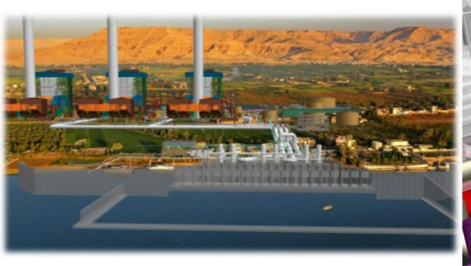
The power block is comprised of three identical Rankine cycle turbine generator units, each with a nominal rated capacity of 650 MW. The units are capable of of both.
